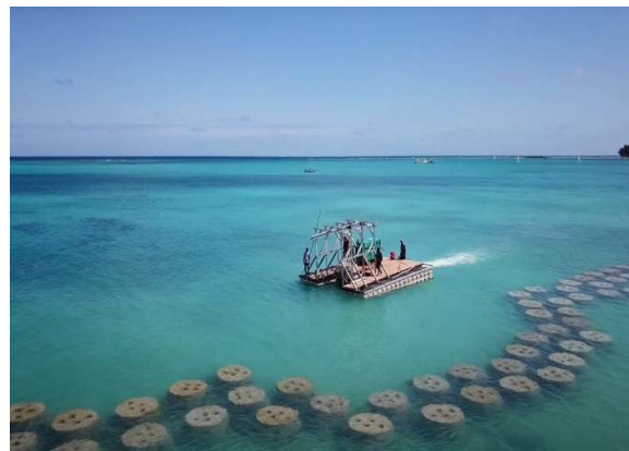
Figure 6 - Installation at Mon Choisy
